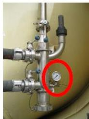
**Step 2:** Start with **building up pressure** by running **compressor** and **opening top air valve**. Also use Aerator from start. Max pressure depending customer.
