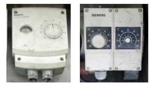
With this type of thermostat, a fixed maximum value is set by the technical department, the temperature set by the driver cannot exceed the fixed maximum temperature.
