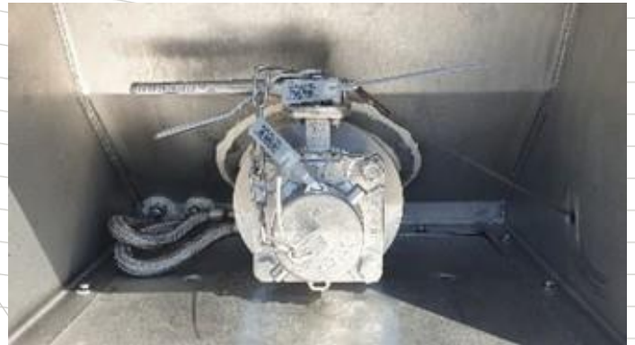
TIR cable sealed to butterfly valve, blind cap sealed
