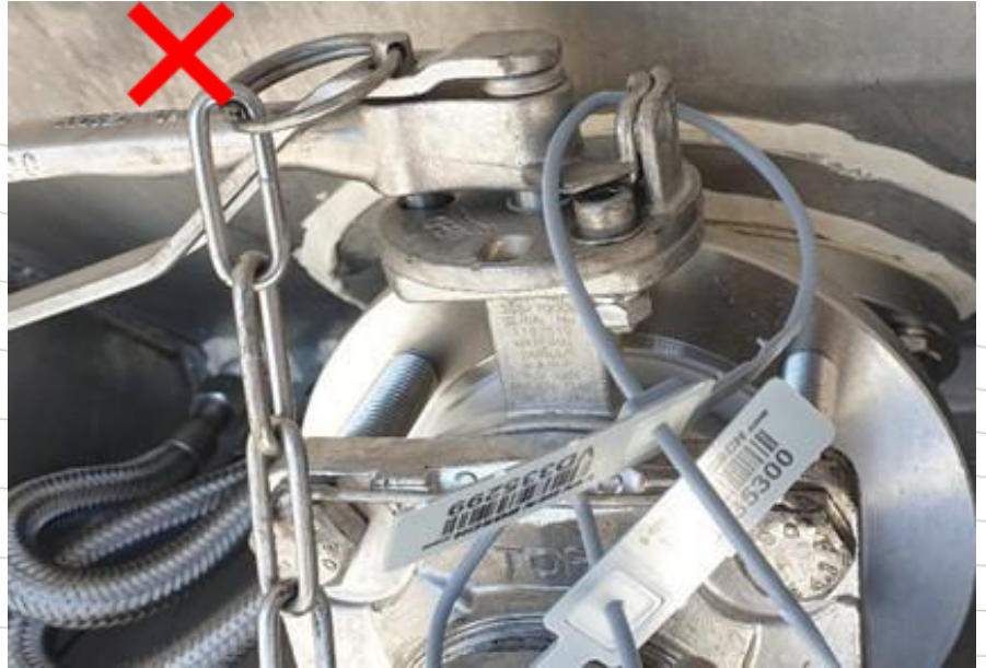
Seal not tightened properly.
